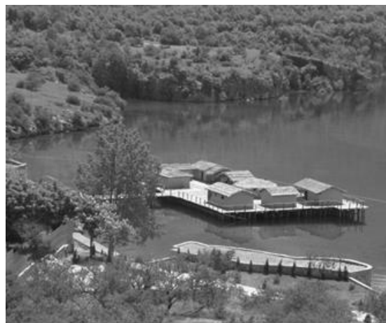
Figure 9. Preview of the authentic reconstruction of timber pile settlement
