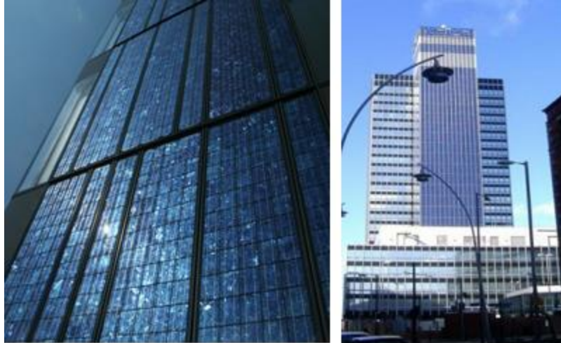
Figure 9. Fasade with integrated PV Panels as Architectural Element
