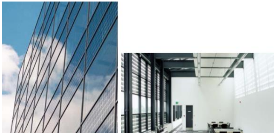
Figure 12. Semi-transparent facade in Office buildings providing sun-light for the workers in the office building
